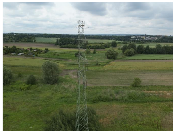
Figure 5. A wide-angle camera view of the surveyed pole, without use of zoom. Shows the actual distance of the drone from an overhead line pole in Chorow, Poland, during trial measurements.
